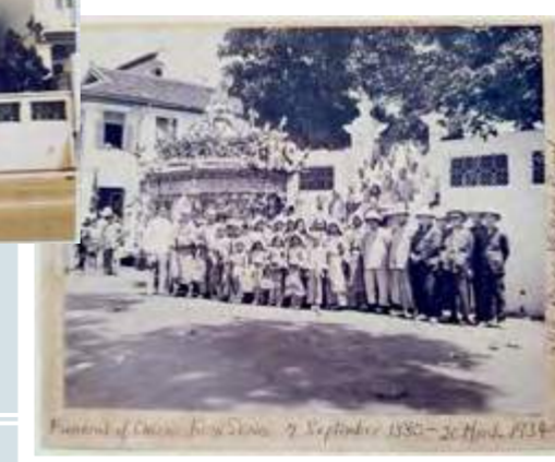
1934 Left | 299 River Valley Road was sold and functioned as Ngee Ann Girls' School until 1981, when the school was relocated to Marine Parade and renamed Ngee Ann Primary School. Right | The funeral hearse of Baba Koon Seng outside his home at 299 River Valley Road. When he died of ill health at the age of 53 in 1934, both ACS and MGS closed for a day to honour him.
