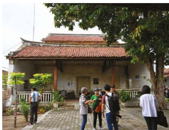
A Chinese-style roof can be seen on the main house in the Lie compound.
